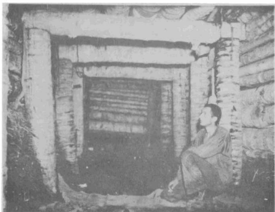
Interior of Japanese bunker.
